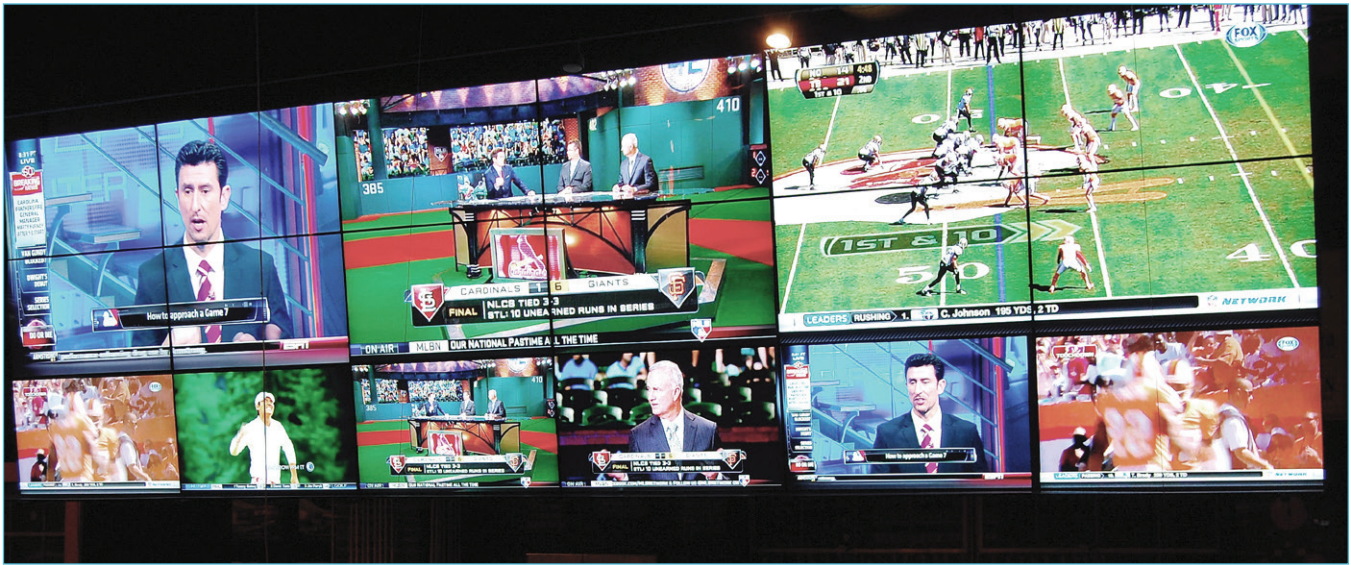
The ultra-immersive video wall captures up to eight cable & satellite set-top boxes and outputs them across 18, 55" displays.
